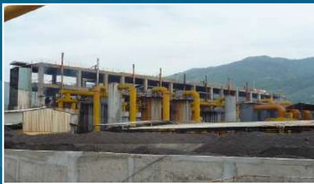
Coal gasification plant, Vietnam
