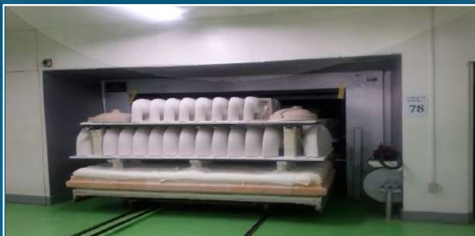
Tunnel kiln, Philippines
